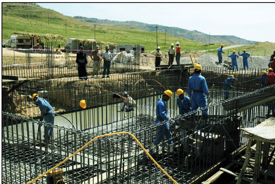
Figure 5-1. An electrical substation outside of Erbil, in northern Iraq. This under-construction substation has eight feeders and two 10-MVA transformers that supply electrical load to three area villages and supply power to local industrial customers. (Photograph by Jim Gordon)
