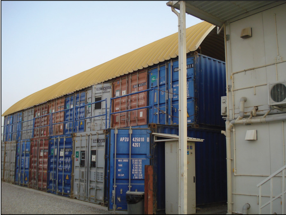
Figure C-2. Intermodal containers altered by bolts, welding containers together, or adding a roof (as seen above) can interfere with the containers' seaworthiness and may lead to complications during turn in. (Photograph by Scott C. Farquhar)
