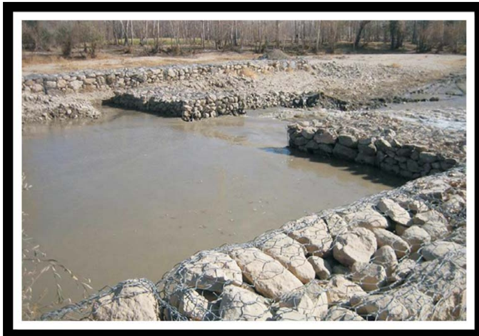
Figure 7-6. Check dam with pooling
