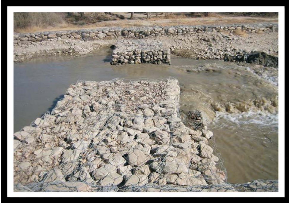
Figure 7-5. Check dam with gabion baskets
